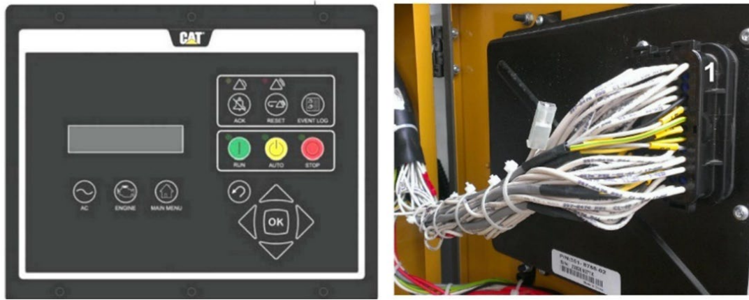
Fig. 33. Main controller of diesel generator
