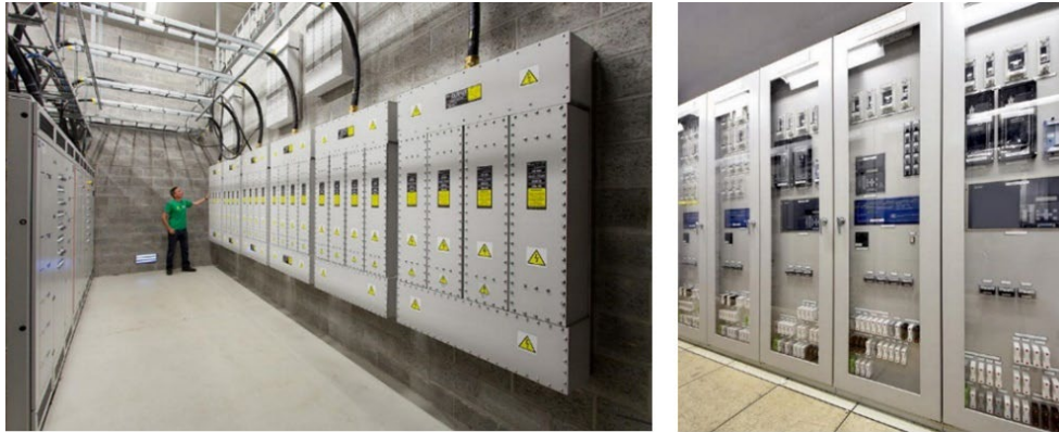
Fig. 12. HEMP filters (left) and control cabinets (right). For size comparison.
